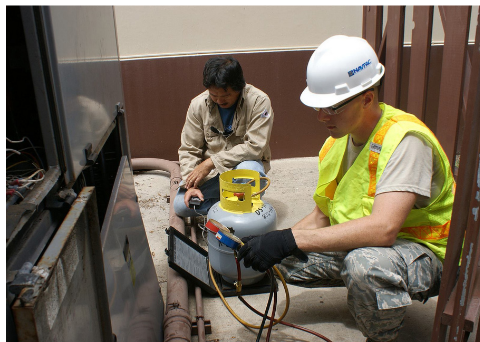
An apprentice working on a HVAC system (Image credit: https://docsavageair.com )
